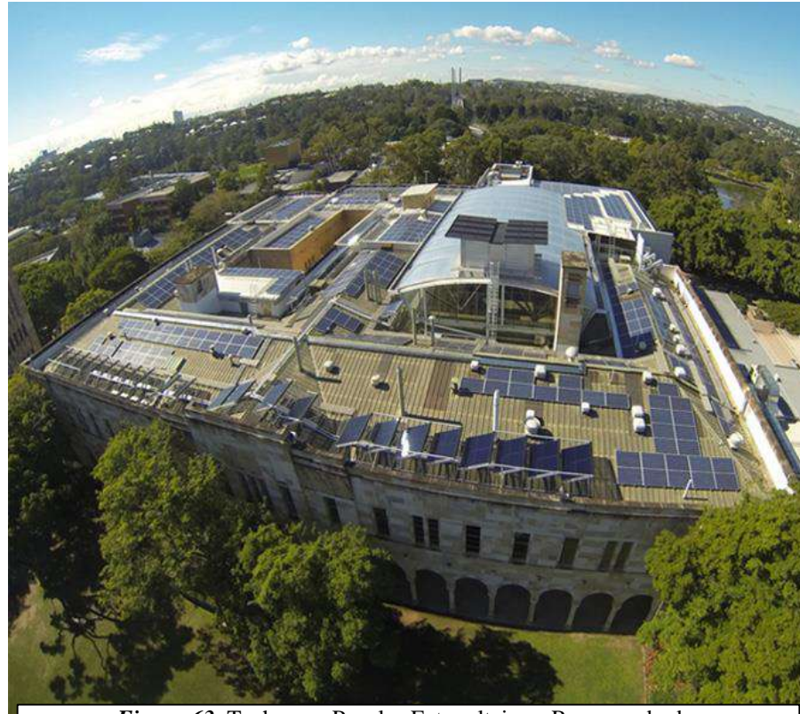
Figura 63. Techo con Paneles Fotovoltaicos. Recuperado de: http://www.mcnab.net.au/latest-news/2016/10/31/video-uq-global-change-institute-building
