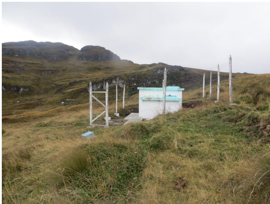
Figura 09: Reservorio sector Chim Chim
