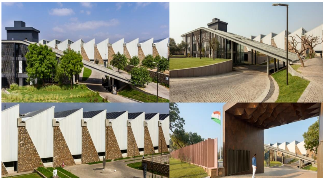
Figura 23. Stonex Industrial Complex.
